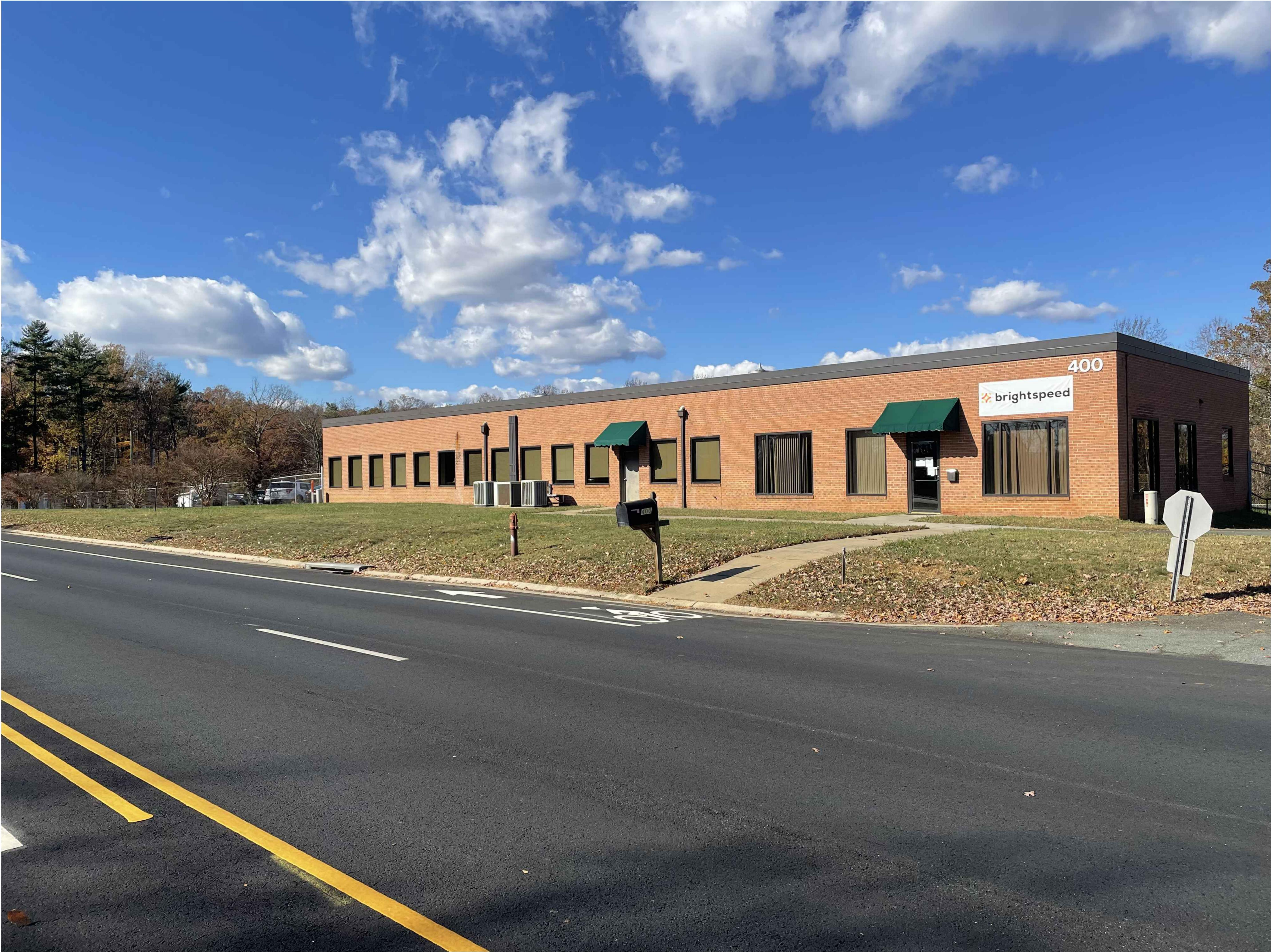
EXISTING FRONTAGE CONDITION - EAST ENTRANCE VIEW
